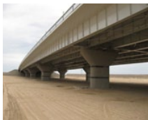
Awaza Bridge (土庫曼斯坦)
